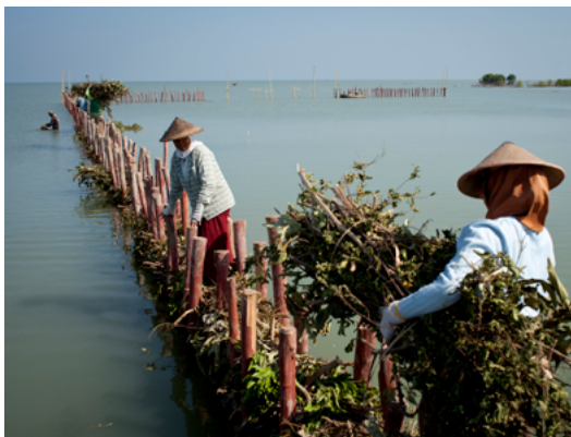
Figure 46: Community groups constructing permeable structures.
