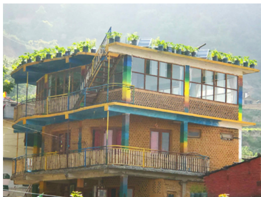
Figure 52: Kindergarten glass bottle and bamboo building
