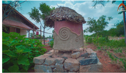
Figure 33 (up, left): Virali ( Dodonaea viscosa ) in cob used as termite resistive admixtures
