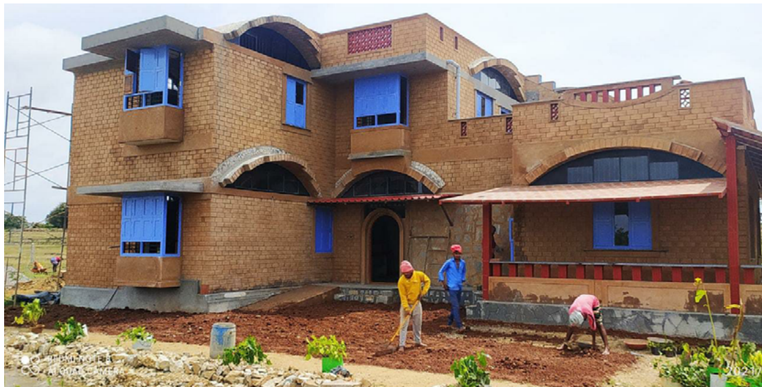
Figure 39: Kitchen garden in the backyard for farming, use of reclaimed doors and windows
