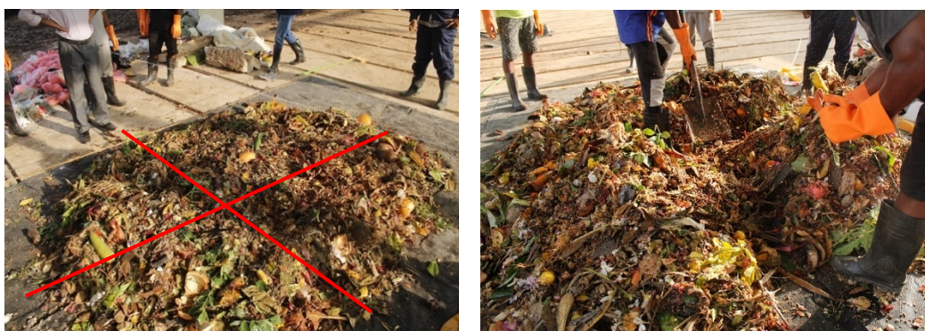
Figure 4: The process of wet waste mixing and dividing into quadrants (Source: WACS Report, 2023)
